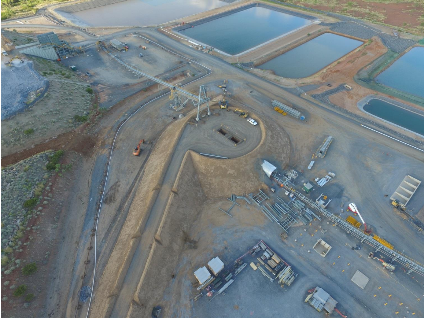
Photo 5 - Reclaim tunnel earthworks
