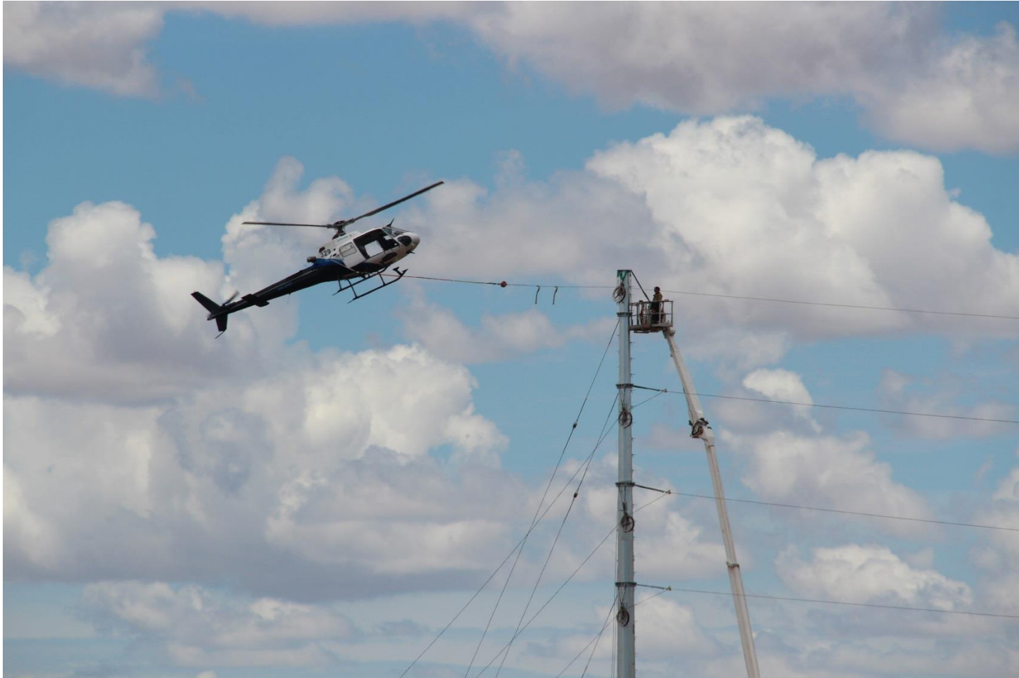
Photo 2 – HV transmission line stringing by helicopter
