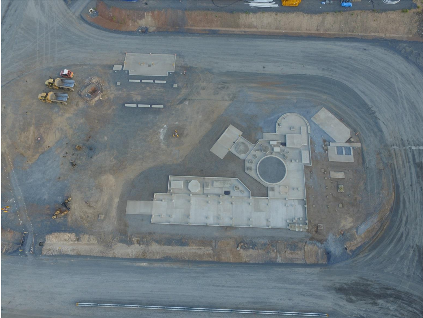
Photo 9 - Paste plant foundations complete
