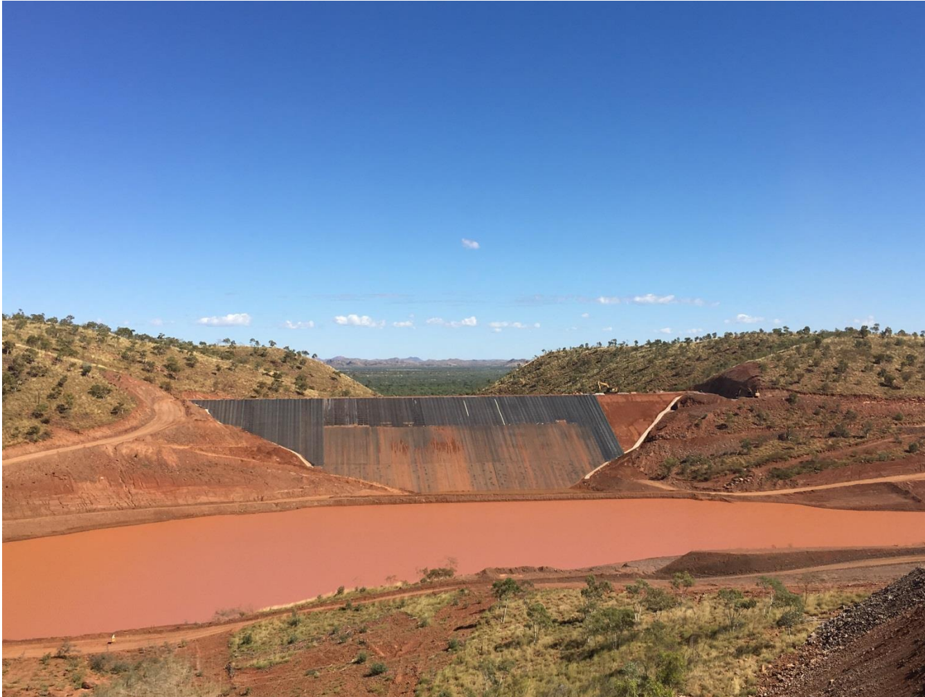
Photo 11 – Tailings Storage Facility dam stage 2 liner installation
