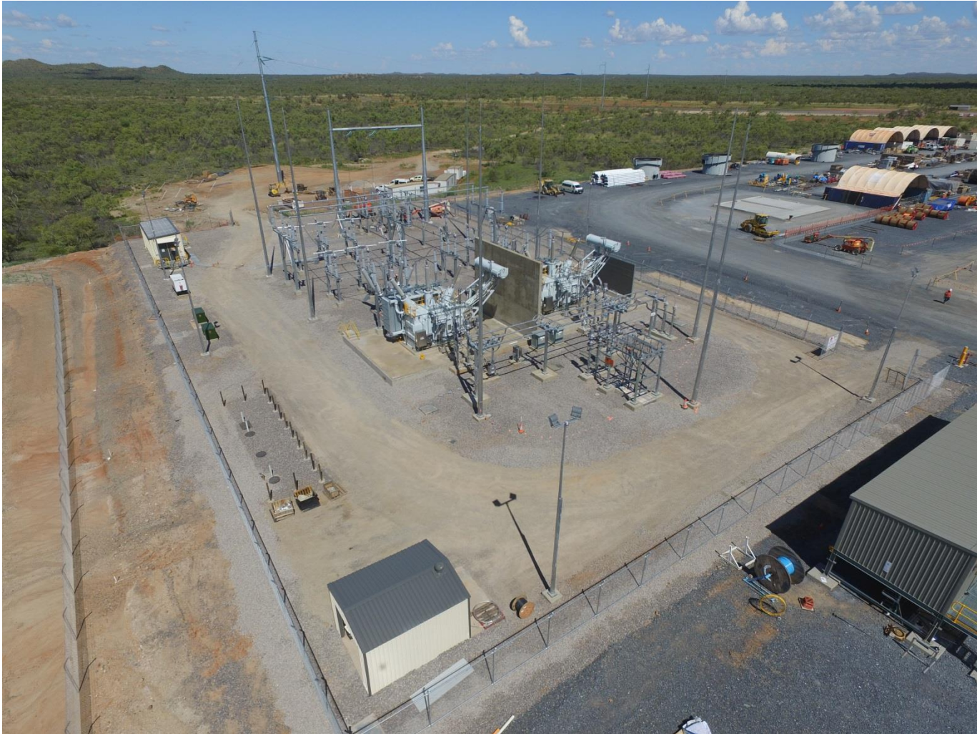
Photo 3 – 220Kv Substation with Transformers
