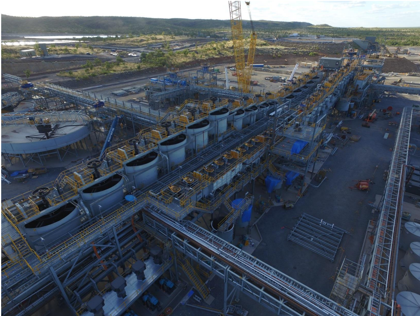
Photo 7 – Process plant flotation cells installed
