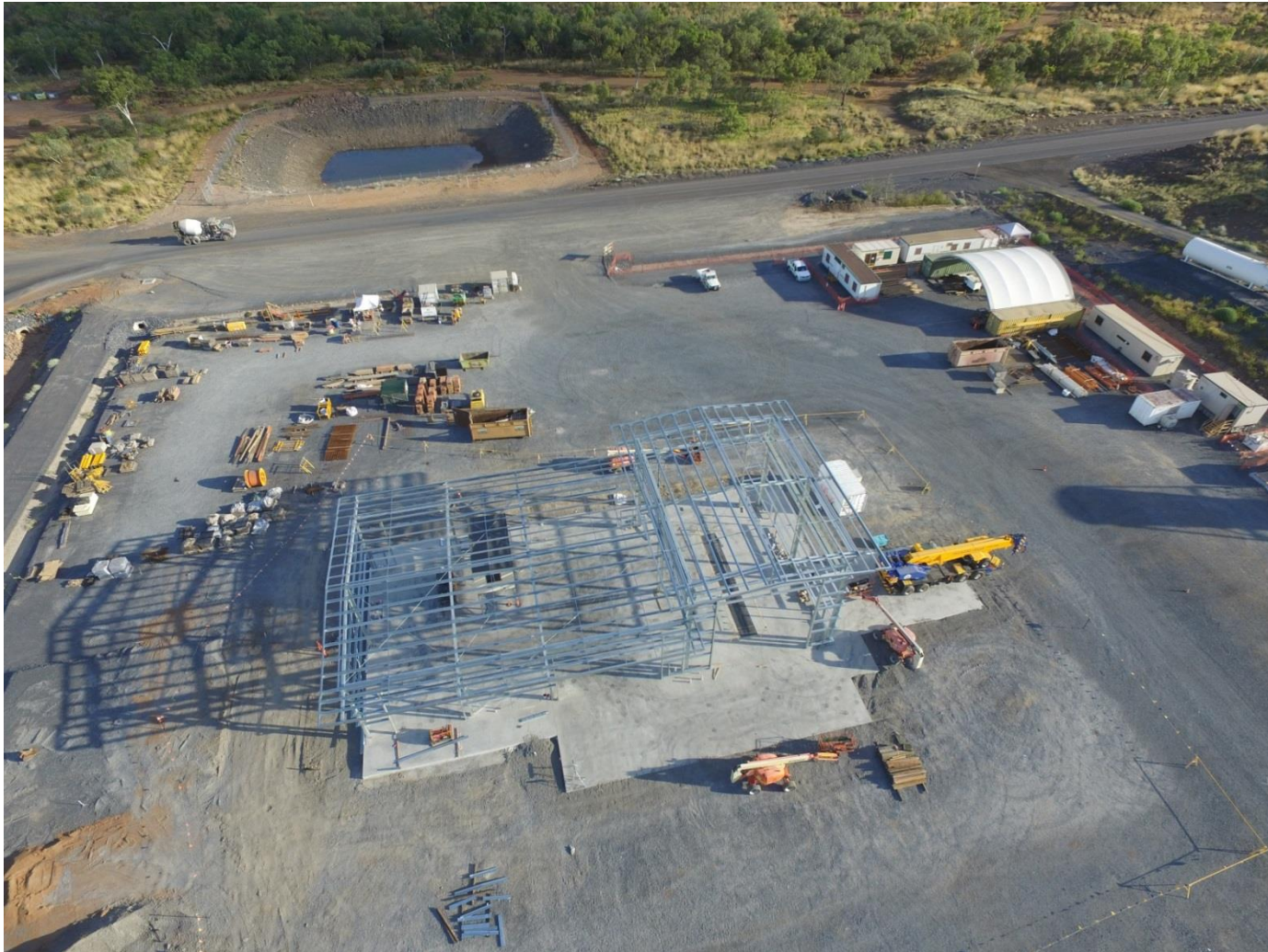
Photo 10 – HV Workshop Structural Steelworks being installed
