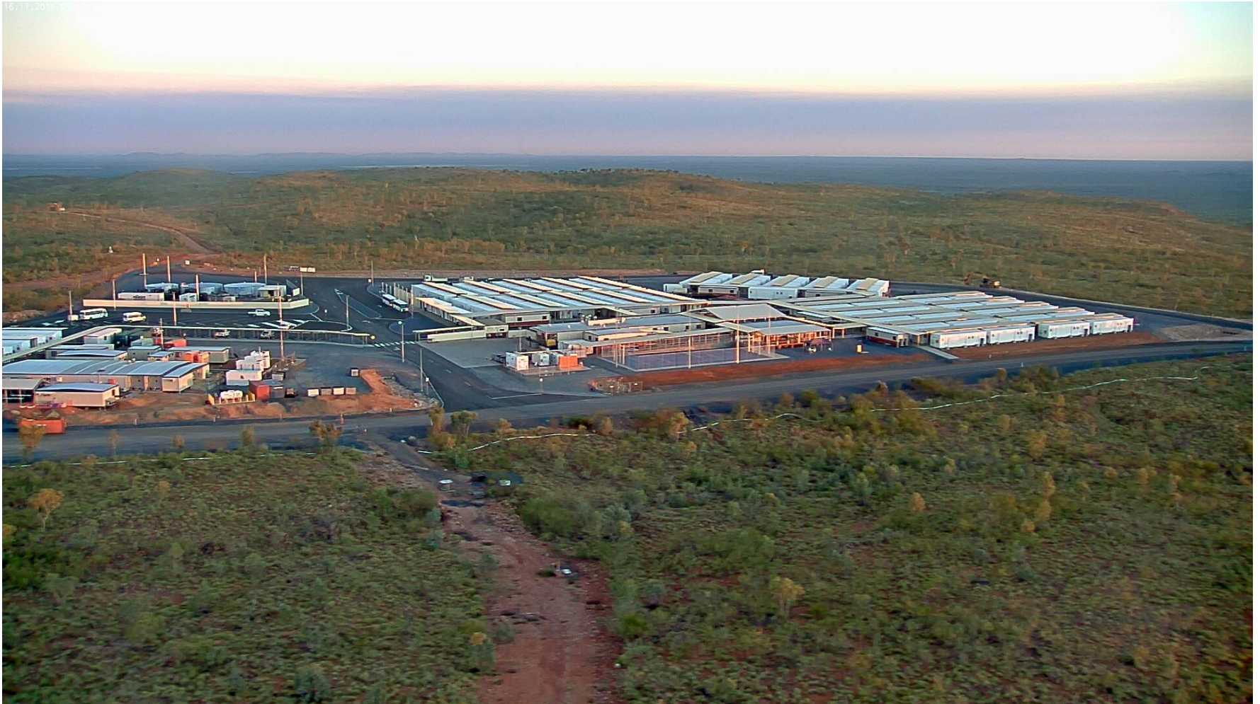
Photo 1 – Permanent Village Accommodation
