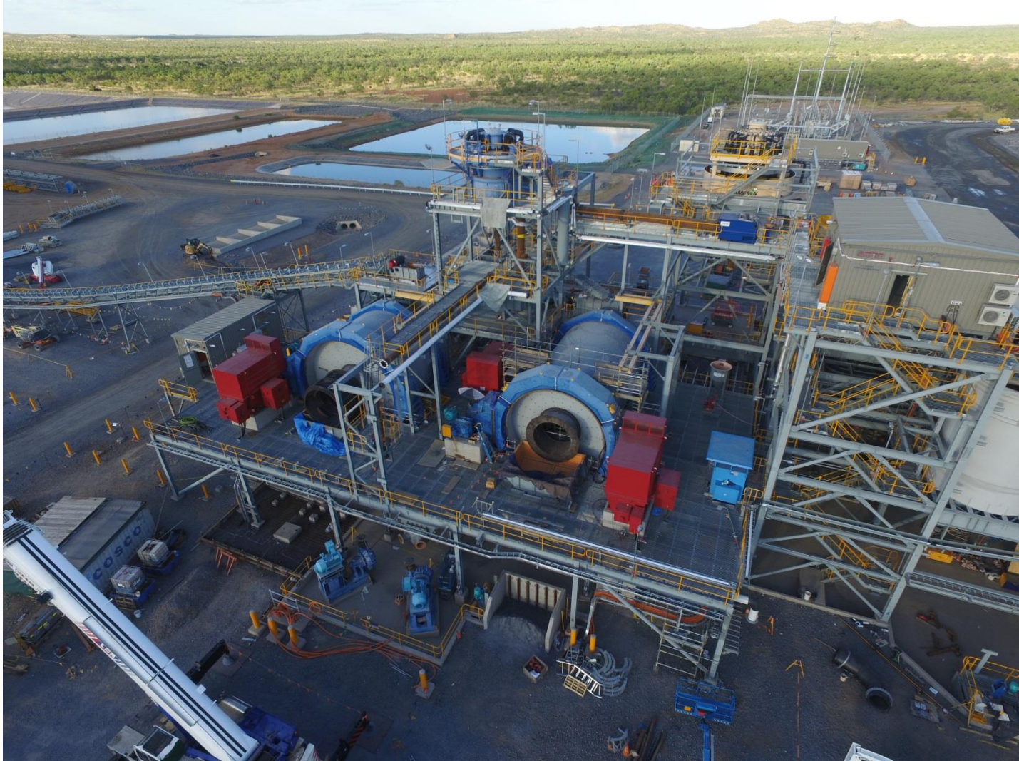
Photo 6 – Ball and Sag mill installed
