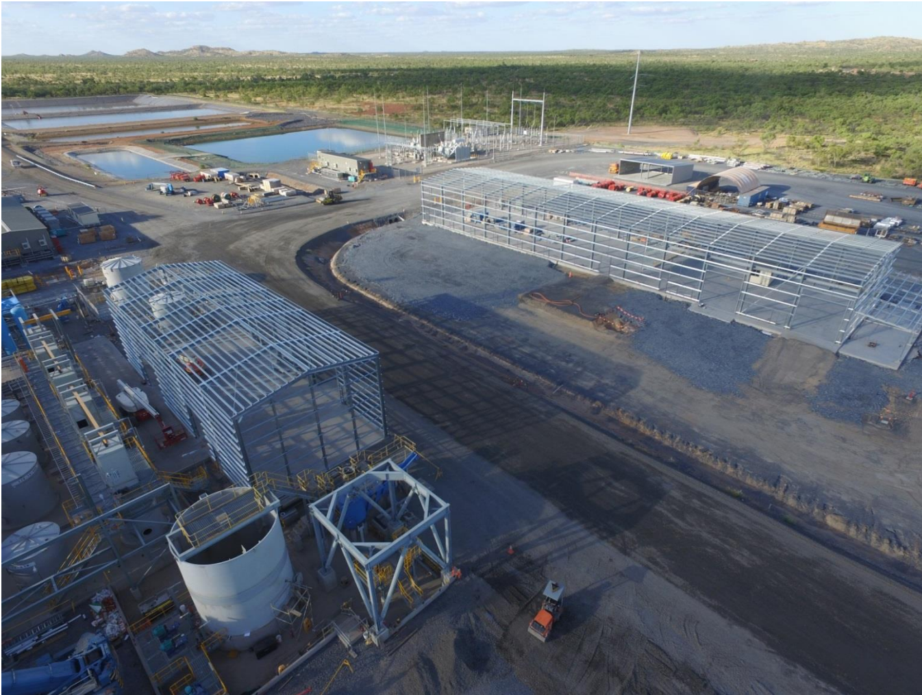
Photo 8 – Reagent building and warehouse structural steelwork installed
